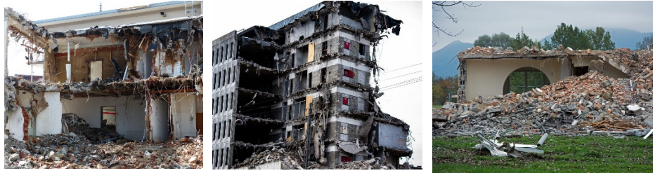
Figure 2 Examples of partially collapsed (2 left images) and total collapse, right
