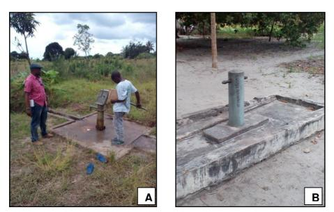
Figure 5-3: Examples of functional (A) and non-functional (B) public water points as found during mapping in Kiromo and Mandawe sub-villages (October, 2014).
