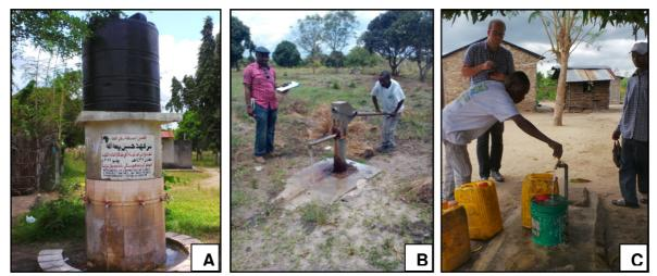
Figure 5-9: Examples of common types of improved water source, a borehole (A), a hand pump (B), and a standpipe (C) as found in Kiromo and Zinga wards (October, 2014).
