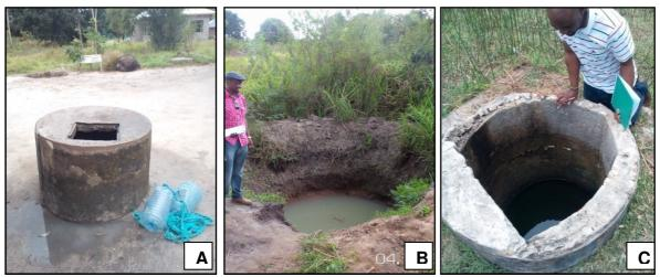
Figure 5-10: Examples of unimproved water sources, unprotected deep well (A), a hand-dug shallow well (B), and open shallow well (C) as found in Kiromo and Zinga wards (October, 2014).
