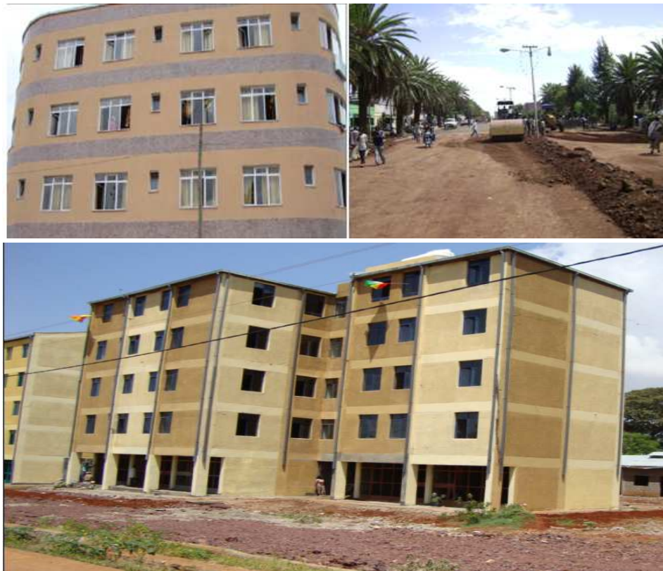
Figure 5.2 Construction activities in Bahir Dar City
