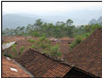
Figure 9-1: Examples of clay tiles roofs in the study area
