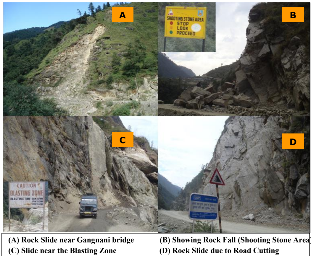
Figure 3-11: Various Landslide Events observed during Field Survey
