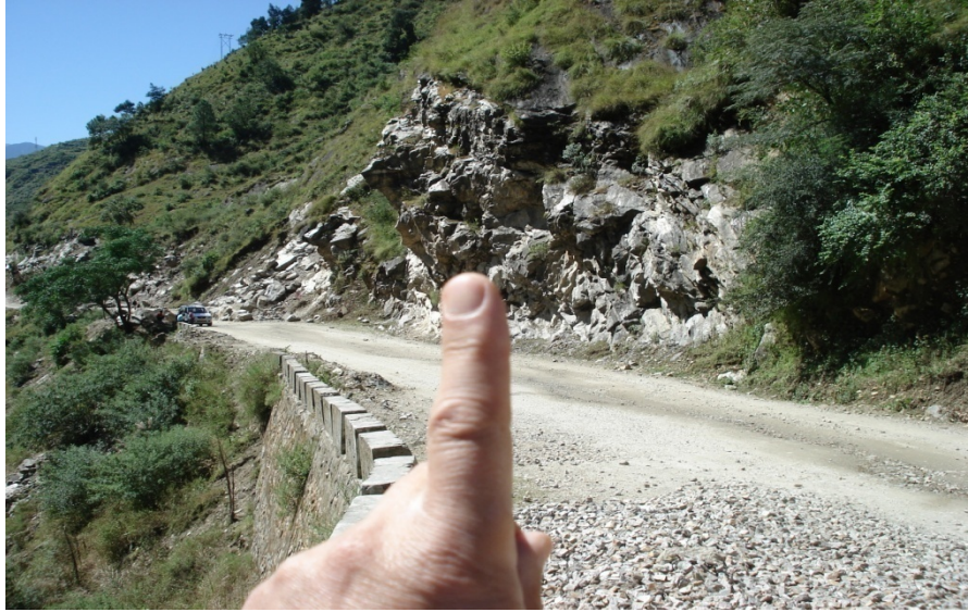
Exposure No-1 near Bhatwari Bridge
