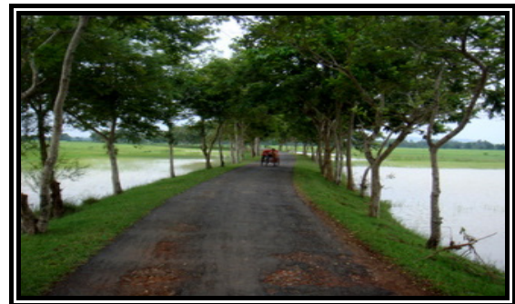
Figure 4-11: Drainage Congestion due to Road
