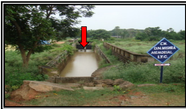
Figure 2-10: Siphon on Birupa river at Triveni
