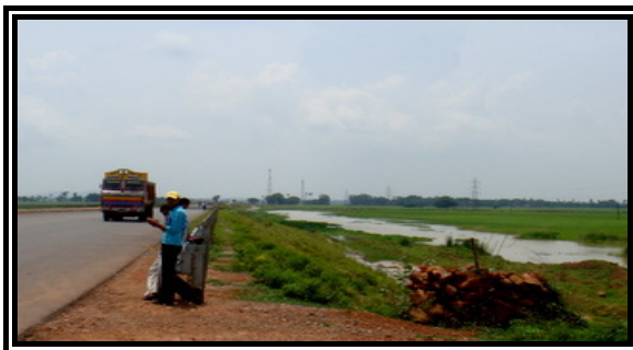
Figure 4-6: Flooded Area along NH 5A
