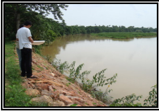
Figure 2-7: Strengthened embankment along Ganguty river.
