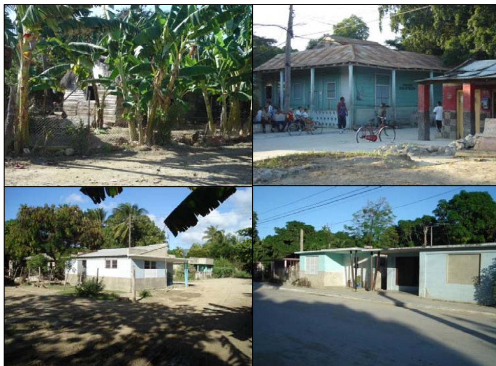
Figure 6.13. Typical houses in San Antonio del Sur. (Clockwise from left to right: wooden house in bad condition, wooden house in good condition, un-reinforced masonry house and reinforce concrete house in good condition (Villalón Semanat, 2007).
