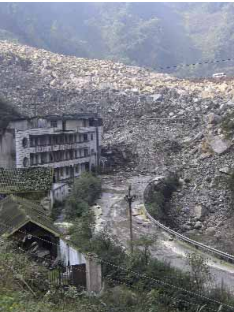
Most of the infrastructure in the area of Beichuan has been lost
