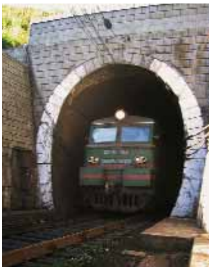
Photo1. Entrance Beskyd tunnel
