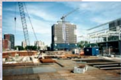
Construction of the underground car park to the north of V&D
