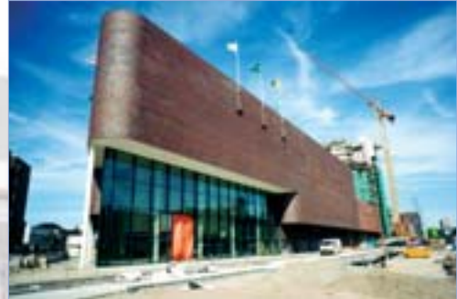
The new casino and shopping centre on the western side of the H.J. van Heekplein
