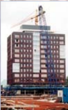
The east tower in the process of refurbishment
