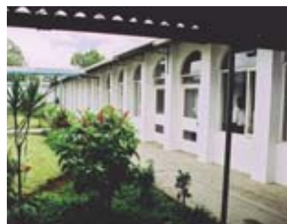
MICOA classroom facilities
