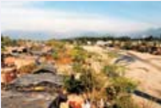
Squatter settlements at risk from flash flood
