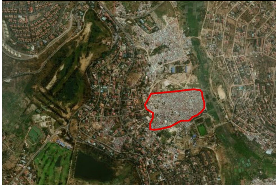
Figure 2.3: Satellite image showing Kangondo II research site to be demolished and redeveloped Source: Esri Imagery, 2018
