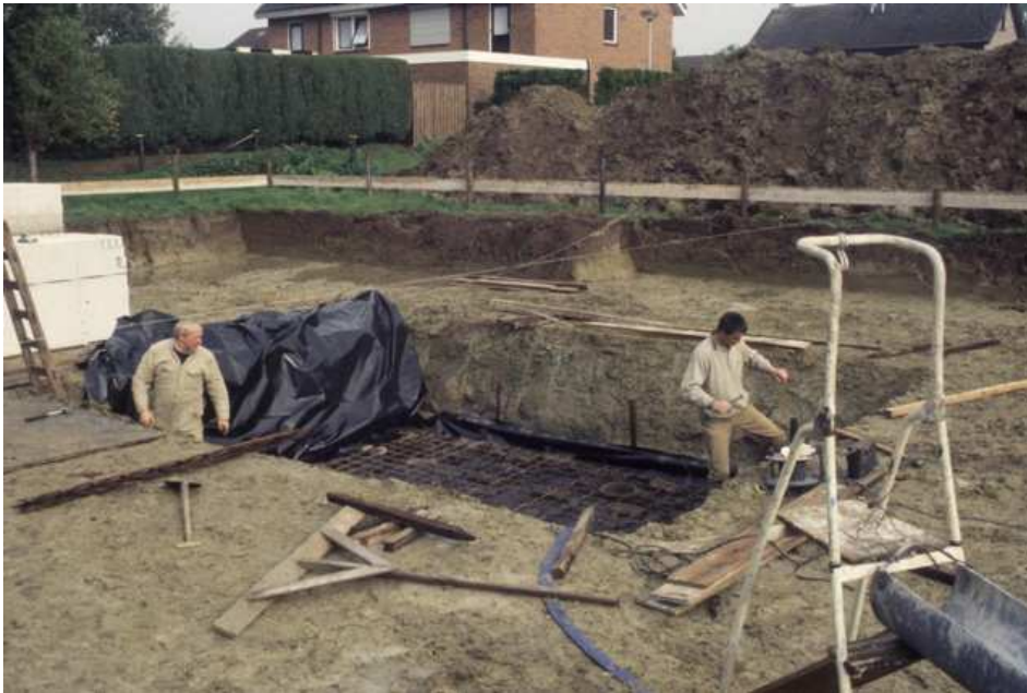
No: house foundation in Tertiary glacially-compacted clay, de Lutte (NL)
