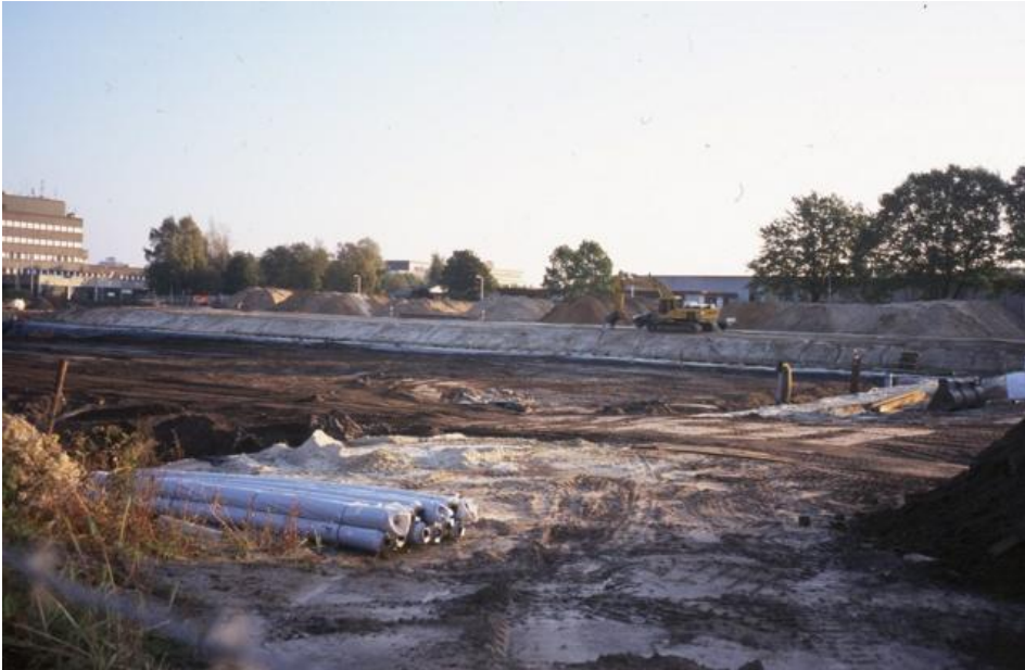
Soil remediation on abandoned gas factory, Enschede (NL)
