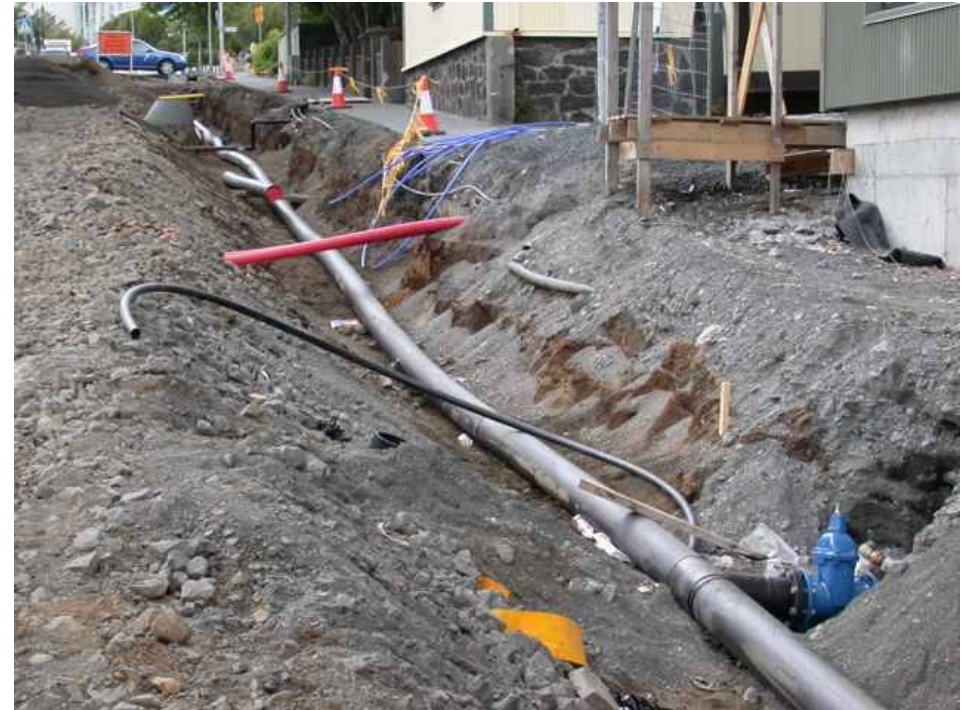
Reykjavík (IS) water pipe; paving
