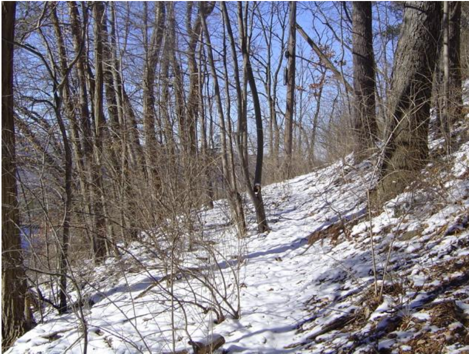
streetcar right-of-way, Ithaca, NY (USA) abandoned for 70 years; frost heave, erosion, colluviation
