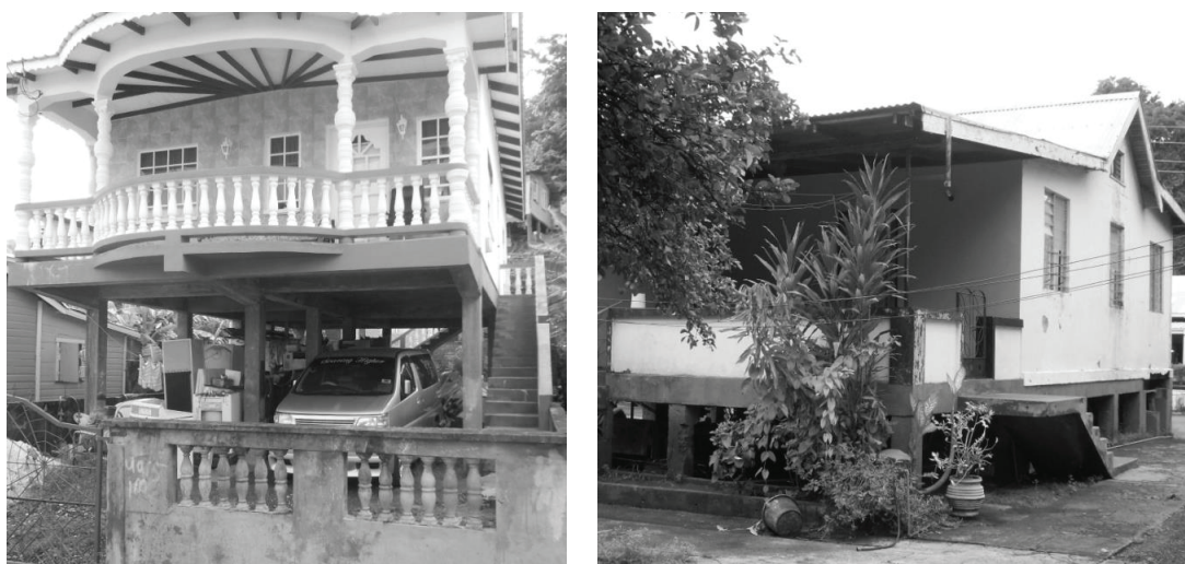
Figure 5.11: (Left) a residential house built top-down (no construction at ground level) in Gonyave watershed. (Right) a residential house built on stilts at St. John watershed, Grenada
