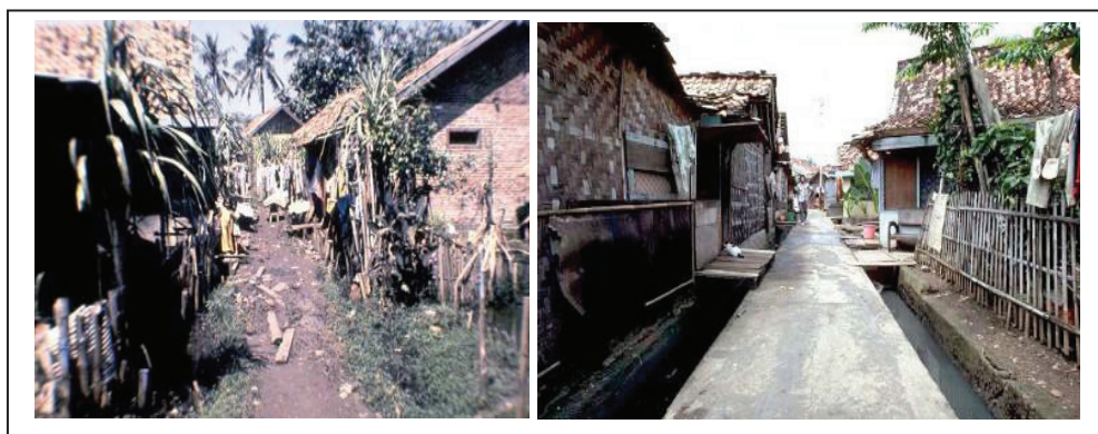
Figure 2-1: Kampung in Jakarta before and after KIP
