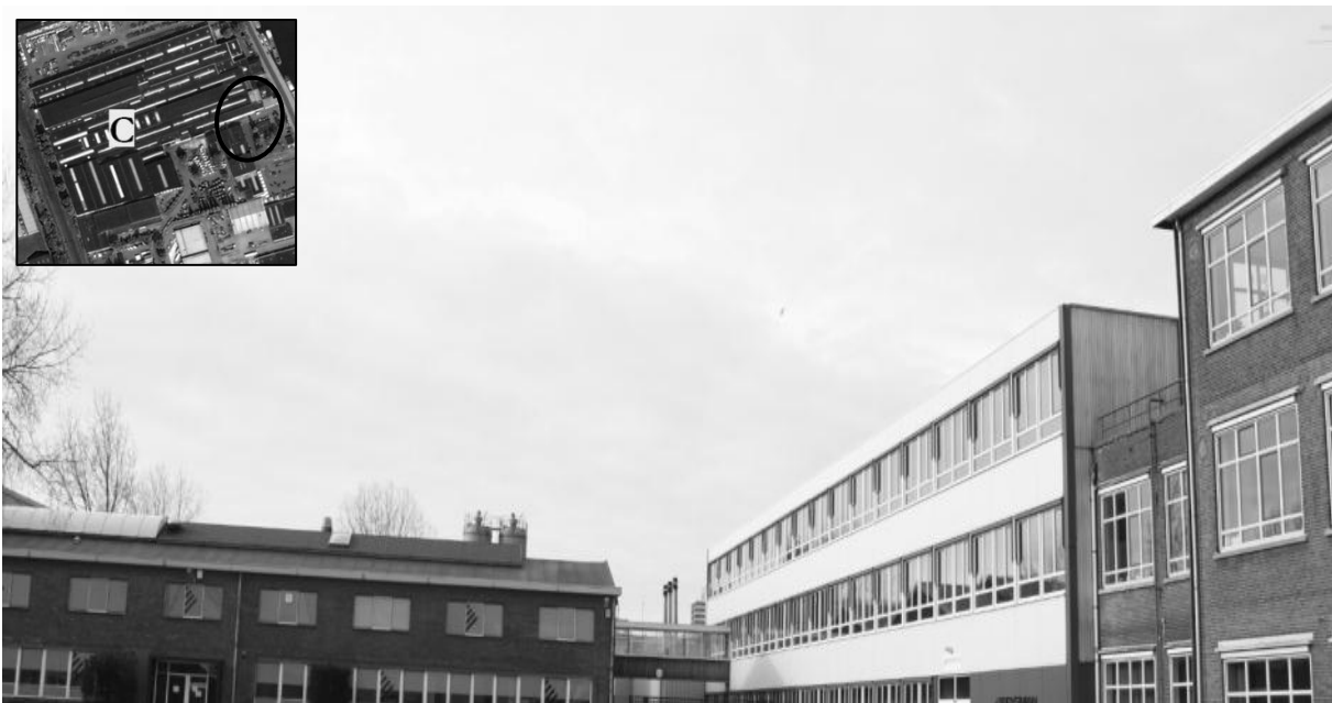
Figure III-2: Building C, study site 2
