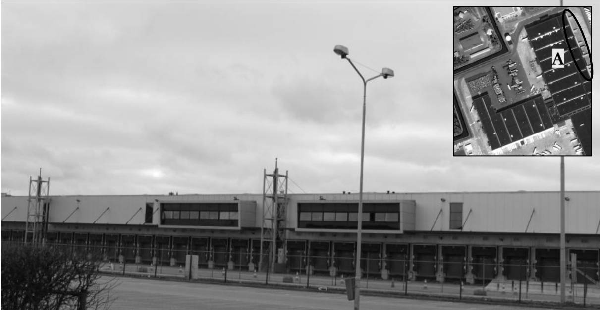
Figure III-1: Building A, study site 1
