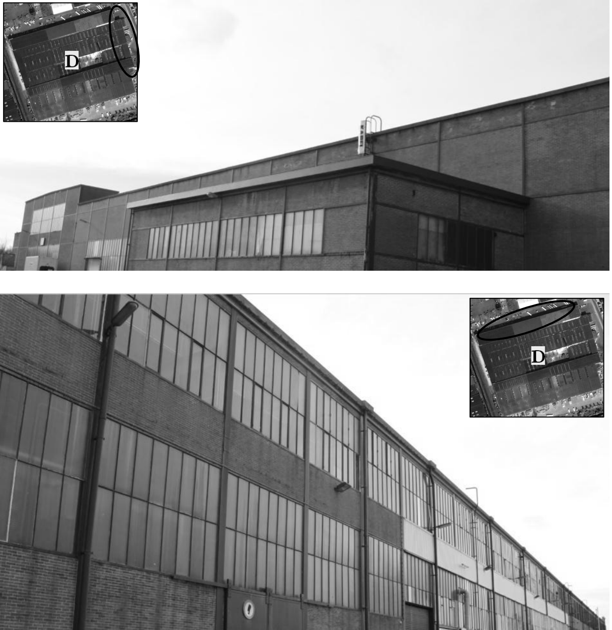
Figure III-3: Building D, study site 2
