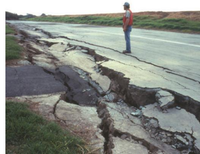
Figure 4: Schematic view and photo of a lateral spreads in California, USA, in 1989 (Highland et al. , 2008)
