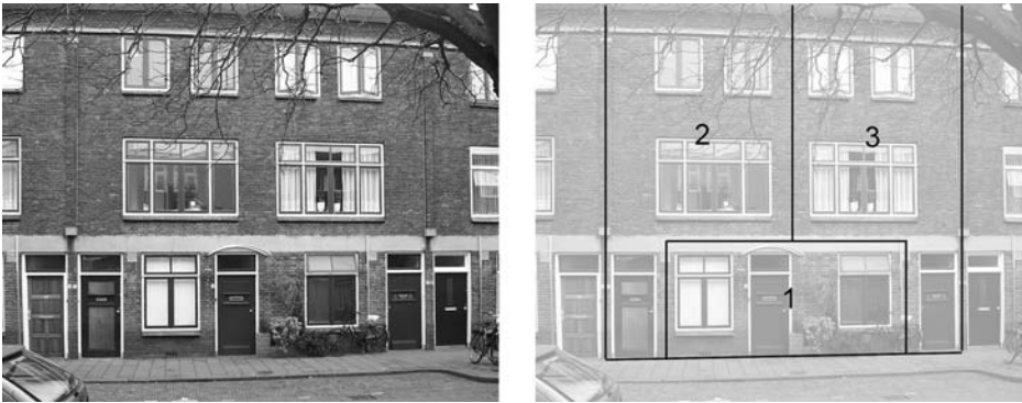
Figure 3.4: Apartment complex used in case study.
