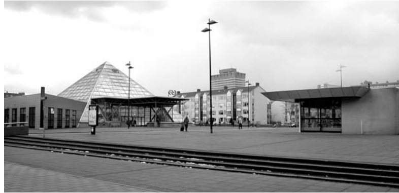
Figure 3.7: Rijswijk railway station (left) and kiosk (right).
