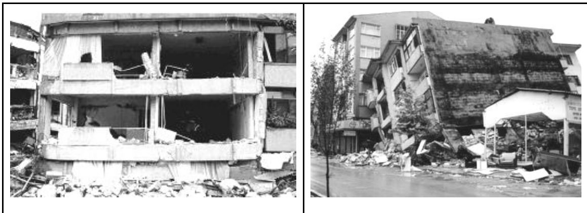
Figure 3.11. Strong beams weak columns (Bruneau, 2002)
