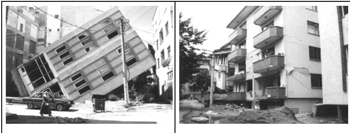
Figure 3.8. Damage due to foundation failure (AIJ, 2000)
