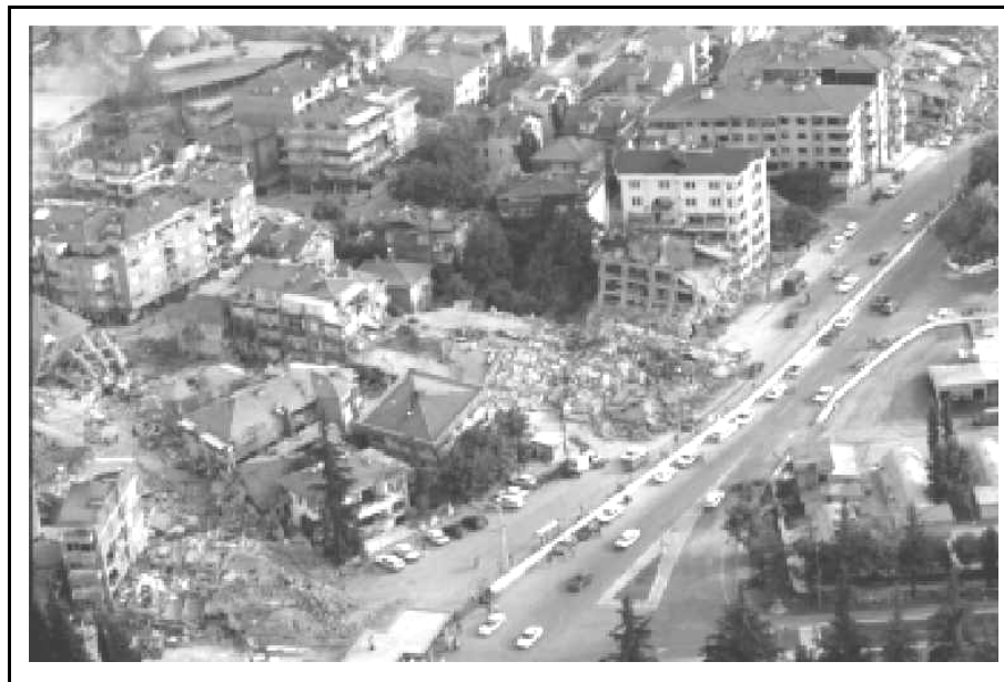
Figure 3.19. A general view of building damage in Golcuk (Erdik, 2003)
