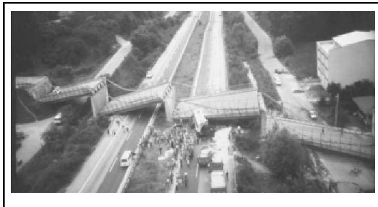
Figure 3.14. Collapse of Arifiye overpass on TEM highway (Erdik, 2003)
