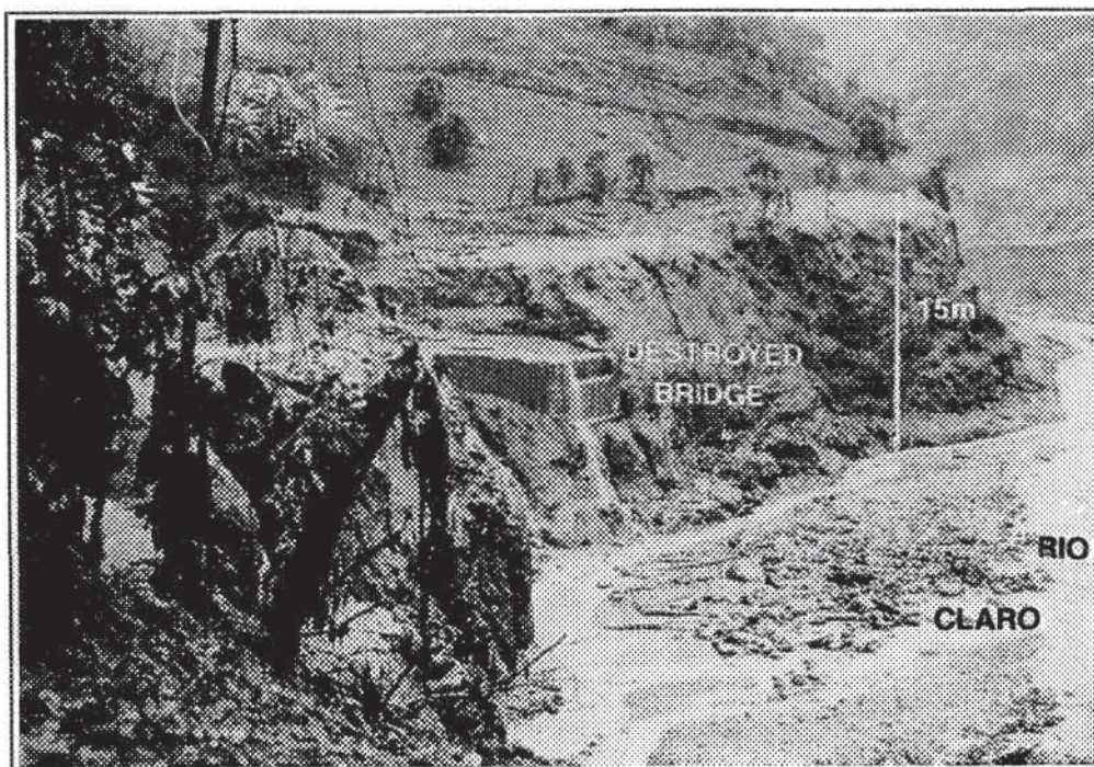
Figure 3.5: Volcanic hazards in the Rio Chinchina catchment. Lahar from 13 November 1985 destroyed many bridges within the Rio Claro valley and reached heights of up to 30 m.
