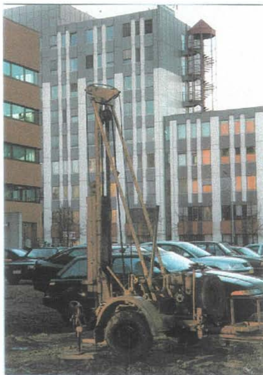
Figure 4.1: Heavy Dynamic Probing test in Maastricht
