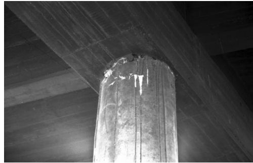
Figure 2.6: Minor cracks on a pillar
