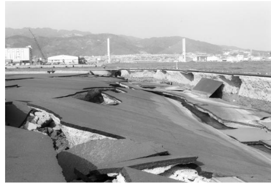
Figure 2.3: Road structure collapses
