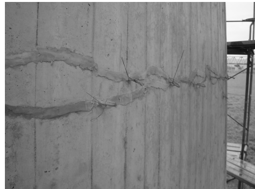
Figure 2.7: Cracks on main support
