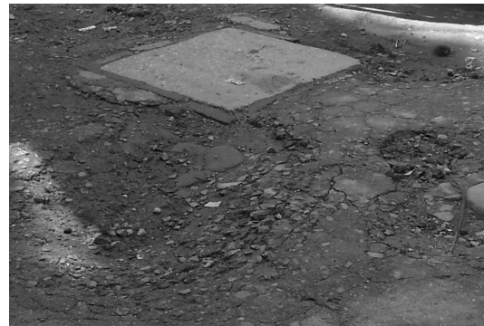
Figure 4.3: Road surface raveling
