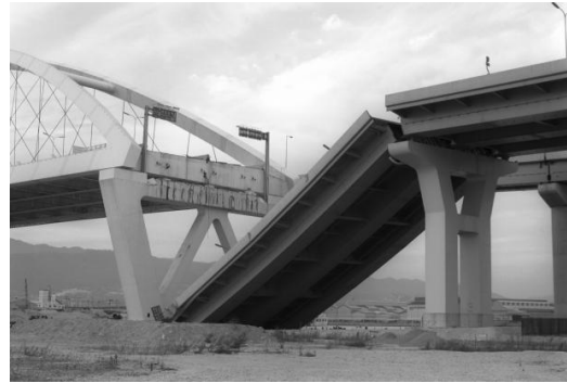
Figure 2.8: Bridge collapsed
