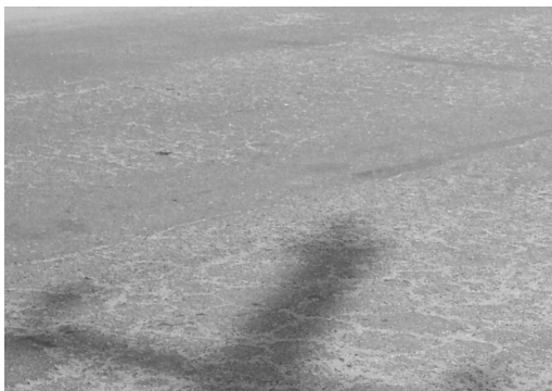
Figure 4.2: Road surface crazing
